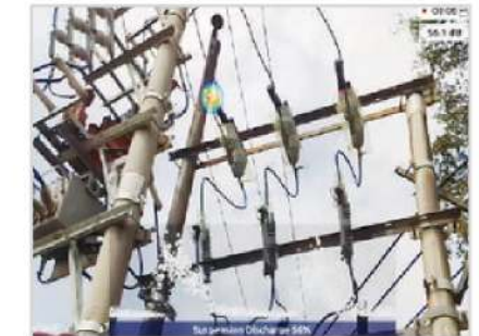
Discharge of 110kv main busbars
