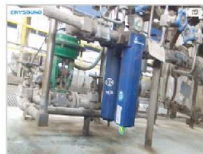
Dry Running gas seals/Nitrogen leak
