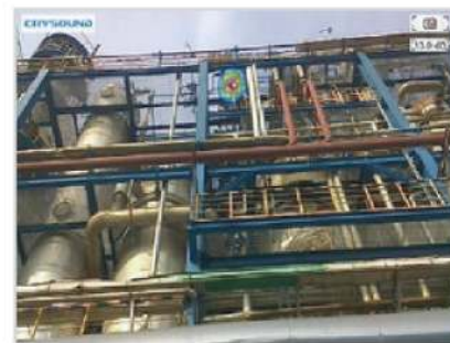
workshop top pipe joint leak
