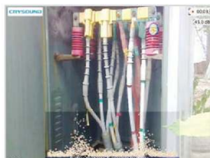
Discharge of support insulators
