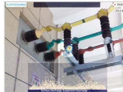
Discharge of insulators on wall-mounted conduits
