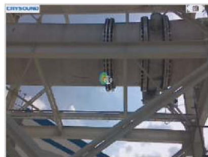
overhead pipe flange leak
